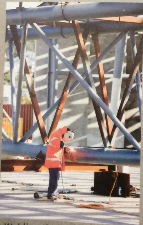
Welding the trusses
