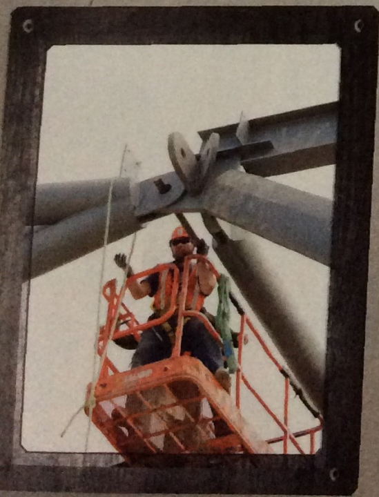
Locking in the trusses
