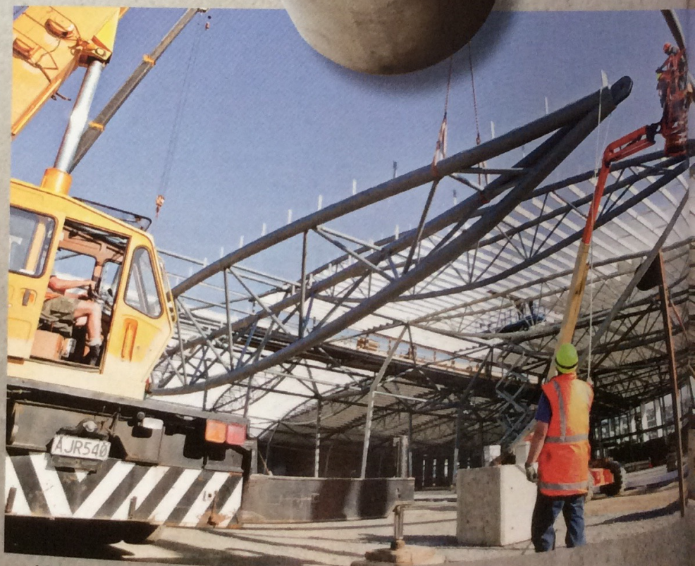
Lifting the trusses
